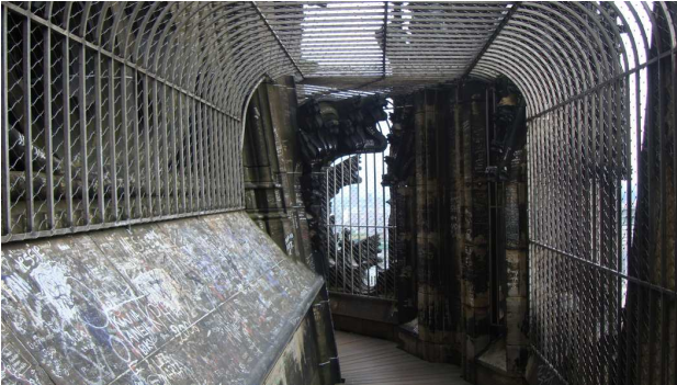
Figure 15: On the top of Cologne Cathedral
