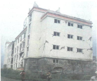
Fig. 9 This building suffered severe damage. The picture presents its north elevation and east of gable wall.
