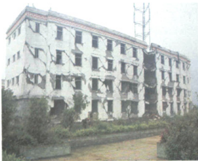
Fig. 8 This building suffered severe damage. The picture presents its south elevation and west of gable wall.
