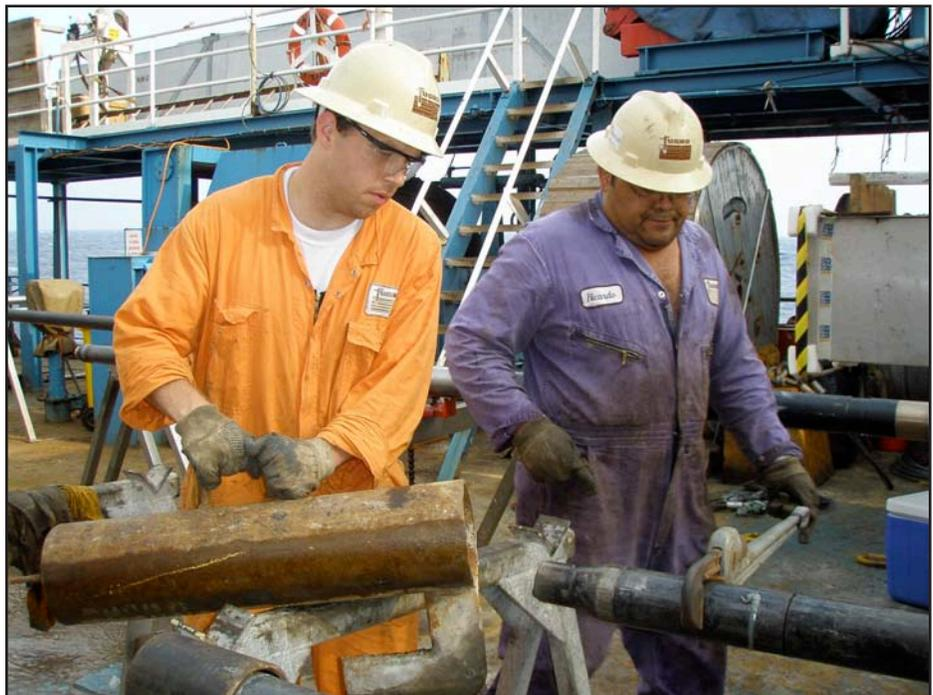
Safety first: the expansive, hydrate-bearing cores must be handled with care. Ben Lunsford and Ricardo Alvarez of Fugro place a safety shoe in front of the corer before removing the cutting shoe.
